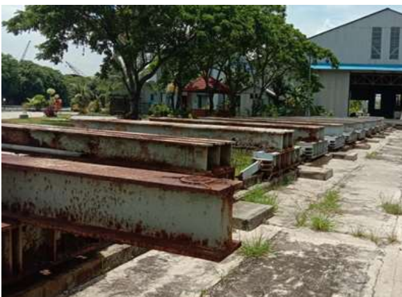
Figure 2. Slipway 750 Tons Fasharkan Jakarta.
