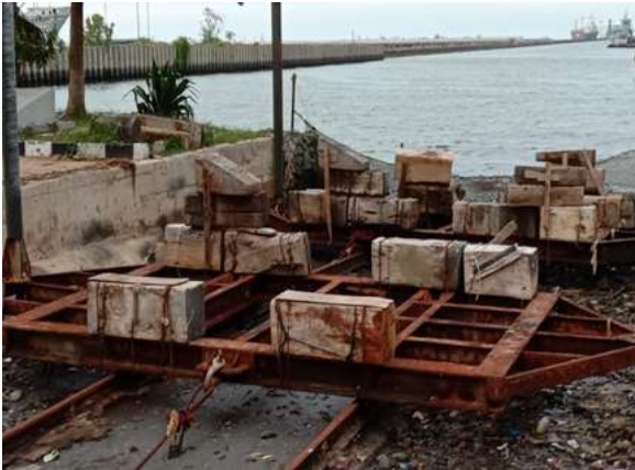
Figure 1. Slipway 50 Tons Fasharkan Jakarta.
