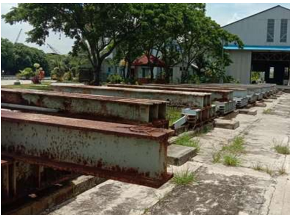
Figure 2. Slipway 750 Tons Fasharkan Jakarta.
