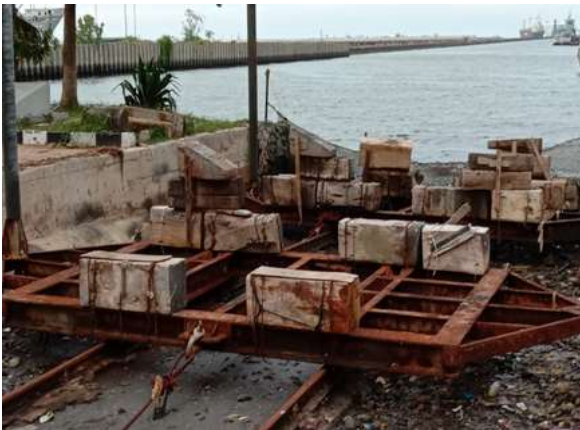
Figure 1. Slipway 50 Tons Fasharkan Jakarta.
